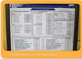
1) Power Meter On-line Monitoring
